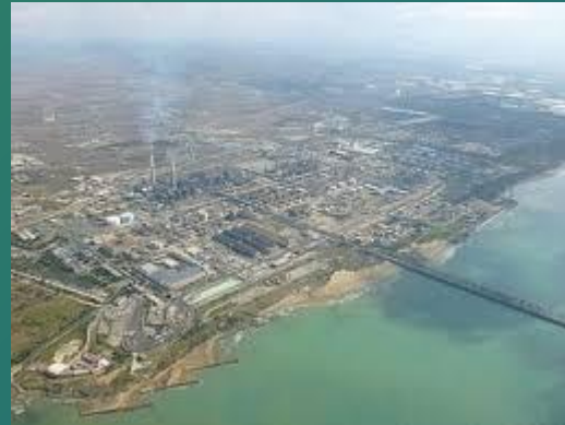
Petrochemical plant – Gela, Italy
